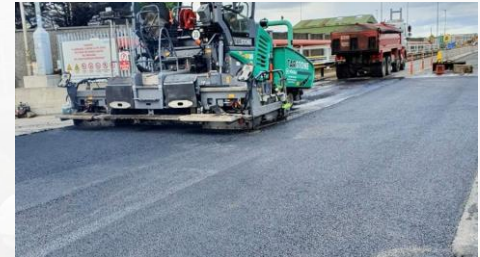
Innovative surface texture with smaller aggregate for increased skid resistance. Active travel schemes.
