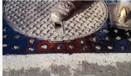
Polymer Modified Mastic Asphalt installation
