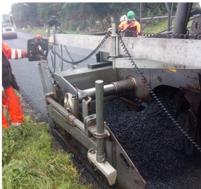
Warm Mix Asphalt
