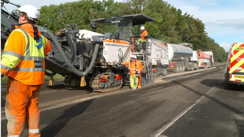
In situ recycling – the down-cut process
